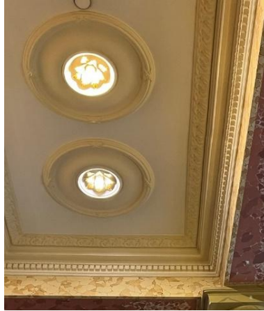
Figure 11. Main Entrance: Coffered Ceiling Detail (Erol, 2022)
