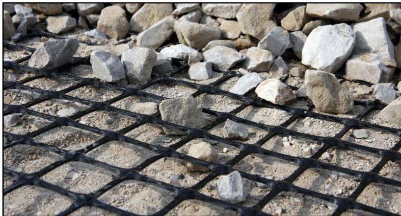
Figure 2.8 Example of Geogrid Utilization URL[1]
