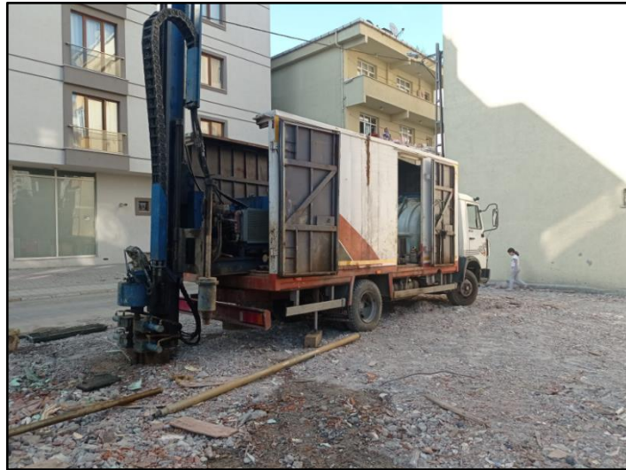
Figure 5.2 The Rotary Drilling Machine Used During The Borehole Operation.
