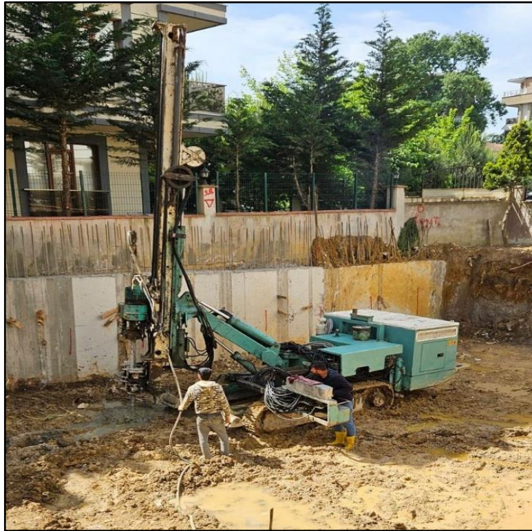
Figure 3.6 Jet Grout Drilling Machine in the Field Environment
