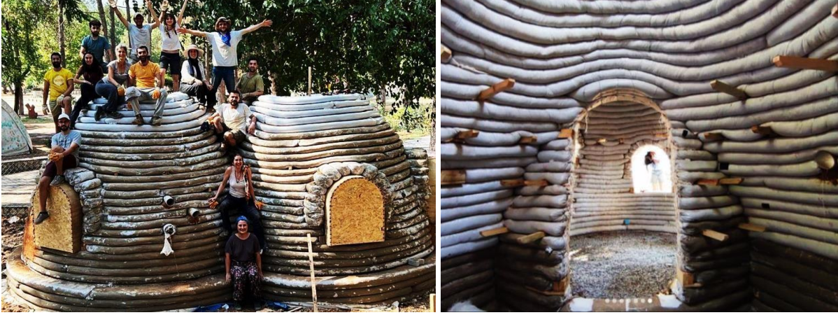
Figure 1. Kahramanmaraş Super Adobe Library project, produced by the Architecture for All Association team, (Xlab, 2023).
